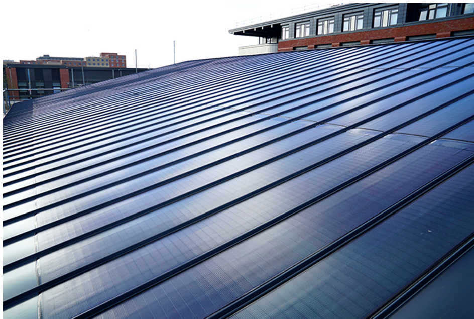
The "Active Classroom" is a zero-emissions building sponsored by Tata Steel built for use at Swansea University near Port Talbot, Wales. Designed for deconstruction, it features the first BIPV Co roof in the UK, made of Tata Steel's Colorcoat Urban steel with integrated solar panels and generates approx. 17 kWp of electricity. It also uses Acermetric Matrix steel-framed panels and Coretinium wall panels. Photo courtesy of Tata Steel.
